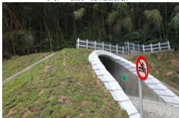
步驟四：假洞口段襯砌及回填
